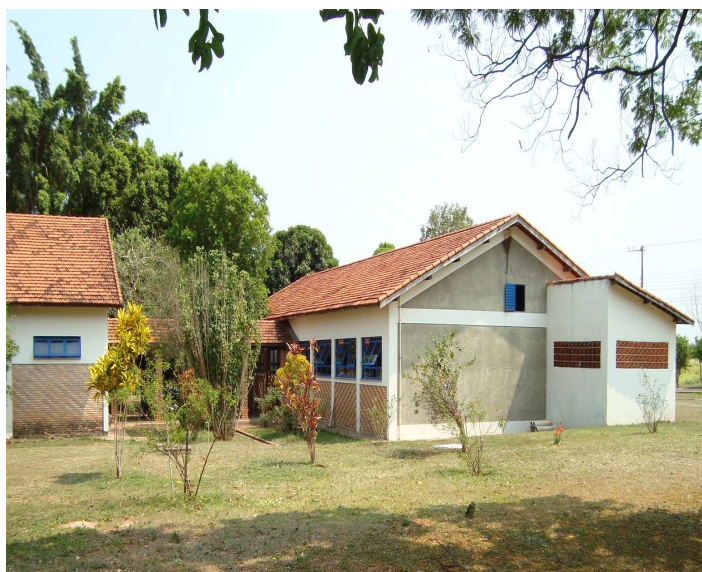
Figura 18 – Bloco perpendicular – entrada principal (UEMS).
