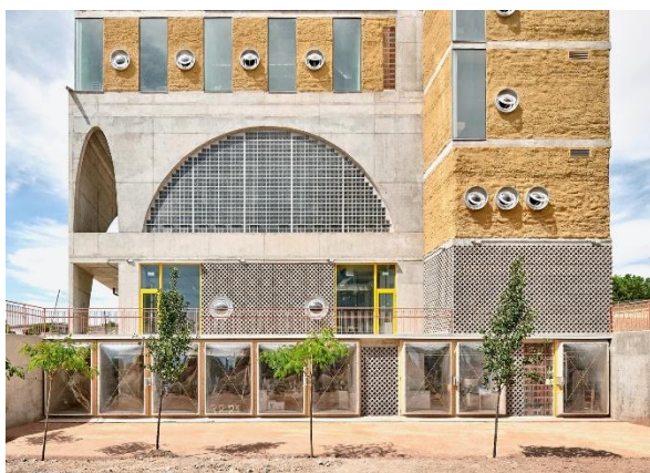
Figura 113 – Colegio Reggio: Fachada Lateral, Madri (ESP) Fonte: Office for Political Innovation, 2022.
