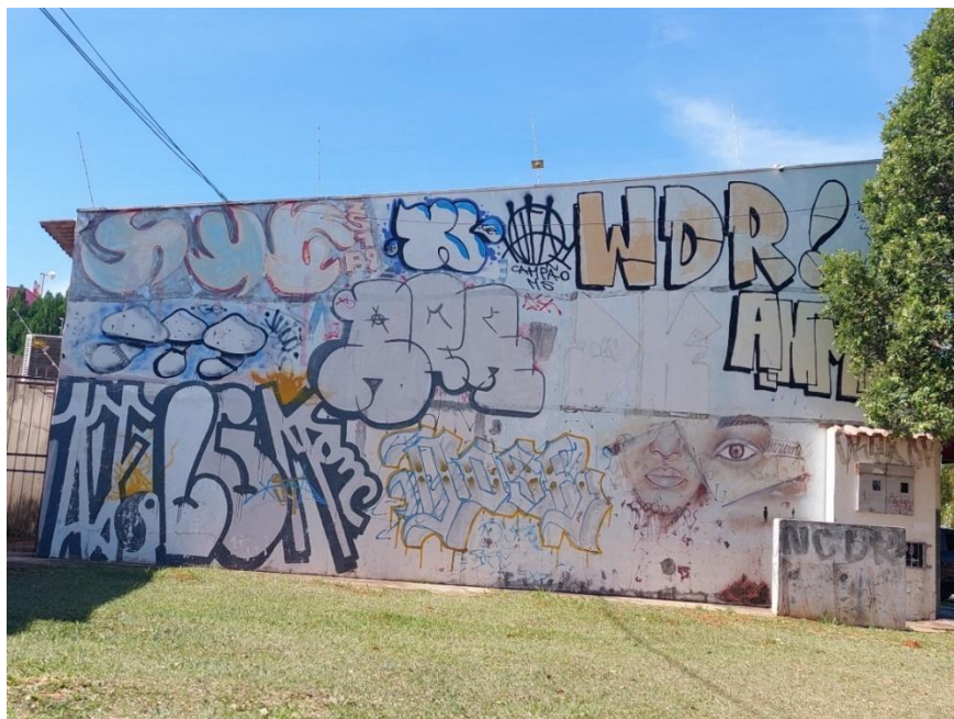
Travessa Camuyrano, Portal do Panamá – MURO RESIDENCIAL – 14/07/2022,10h13
