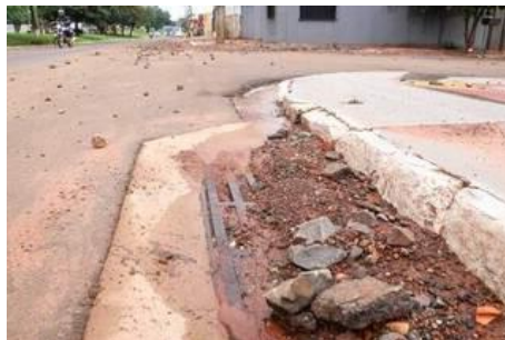
Fig. 9 Obstruction of storm drain at Segredo UHM
